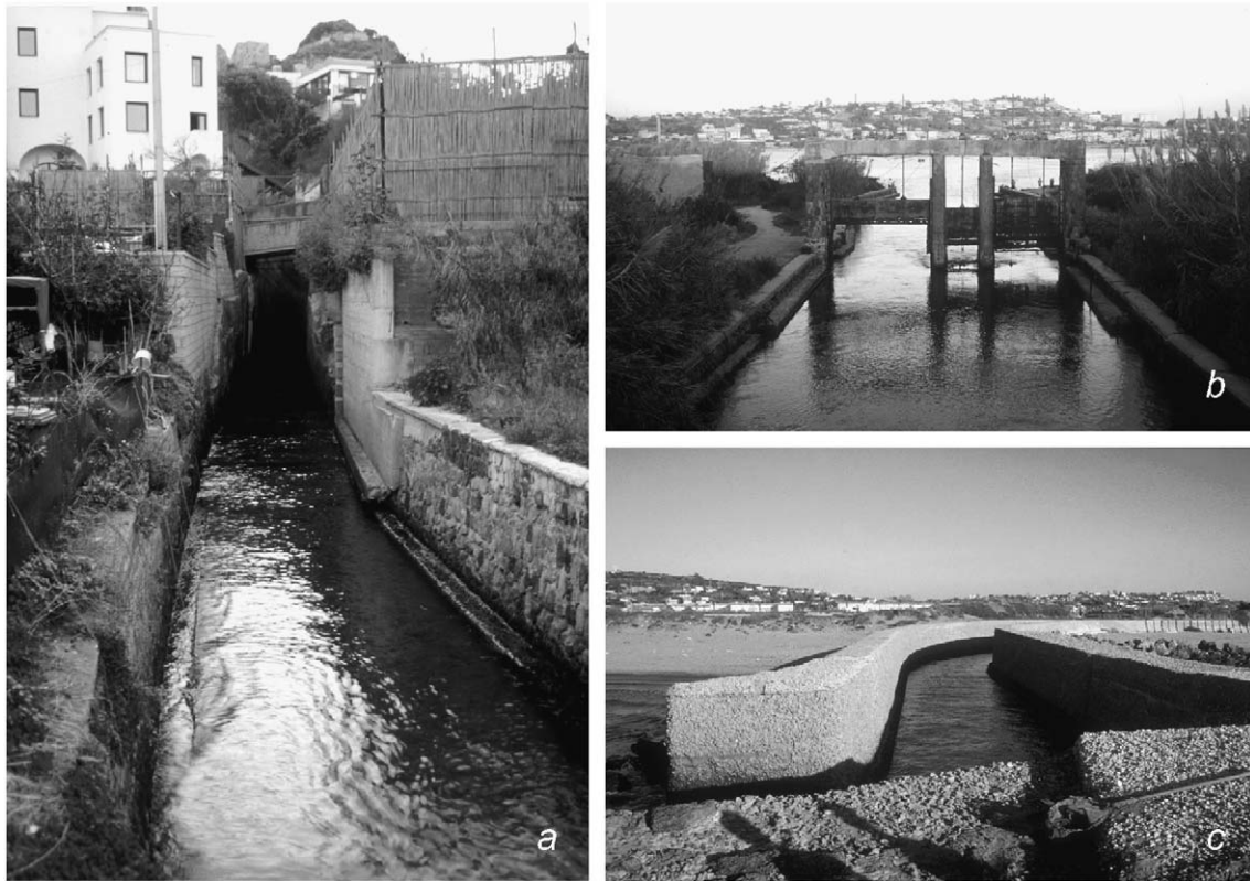
Fig. 3. The three artificial channels which connect the Fusaro Lagoon with the sea. (a) Foce Vecchia channel, constructed in the Roman period in the southern area cutting through a channel in the tuff. (b) Foce Borbonica or Nuova channel, located in the northern area and constructed in 1859. (c) Foce Centrale or di Mezza Chiaia channel, opened between the other two channels in 1941.
