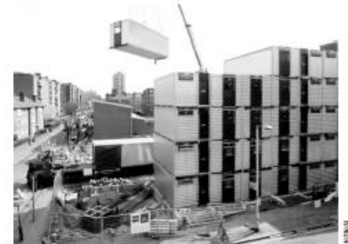
Murray Grove under construction
